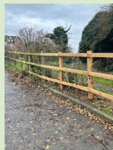
After - New rail and post fence to replace broken section
