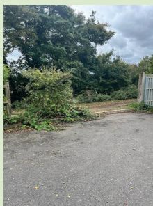
Before - broken fence
